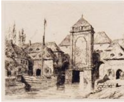
TOURNAI Bridge and Water-Gate
